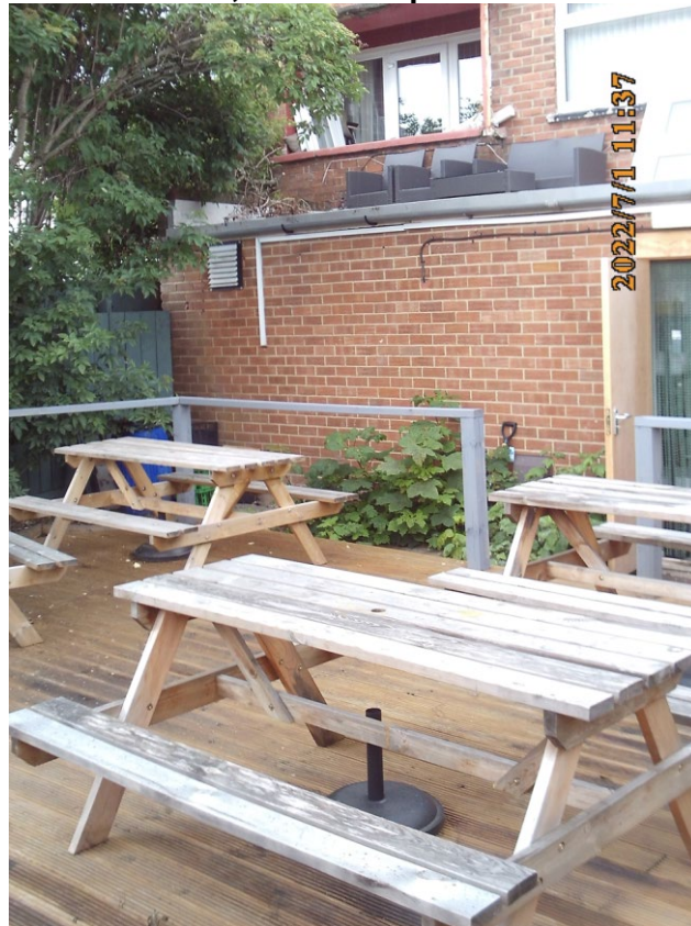
Photograph One: External Area, flat above premises overlooking external area.
